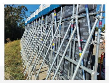
1. SafeSmart designed, engineered and supplied a 3-metre high noise wall, approximately 160 metres long utilising Proscaf sub-structure bolted to the capping beam on site.
