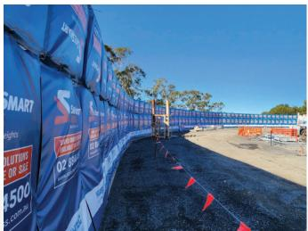
2. The second involved designing and supplying a 17-metre retractable acoustic curtain that spanned across the site driveway. The acoustic curtain was assembled and disassembled daily to accommodate the proposed night works.
